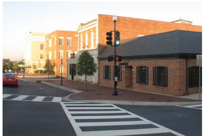
This intersection at Morgan Square contains several outstanding design features such as high-visibility crosswalks, pedestrian signal heads, pedestrian-scaled lighting, and ADA-compliant curb ramps that make the intersection safer for pedestrians and vehicles
